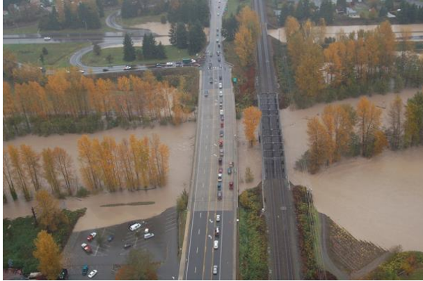
Figure 6.25. Flooding November 7, 2006, SR 410
