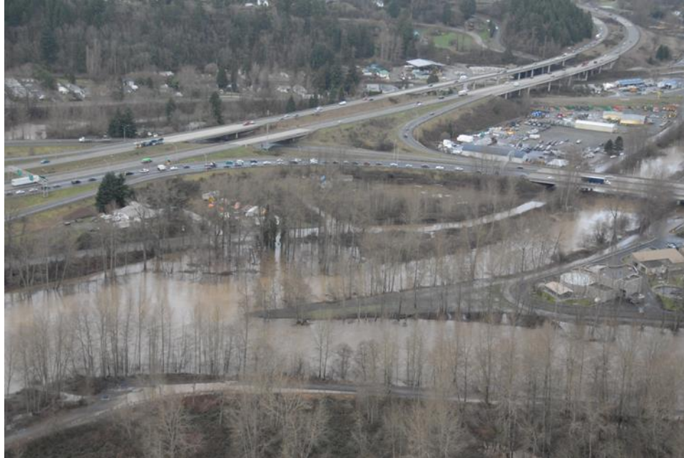
Figure 6.17. Flooding January 8, 2009, Houston Road East
