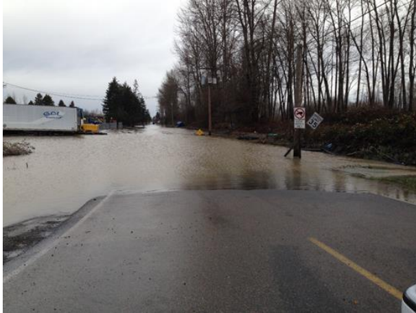
Figure 6.53. Butte Avenue during a High Water Event, December 2015 (Looking North)
