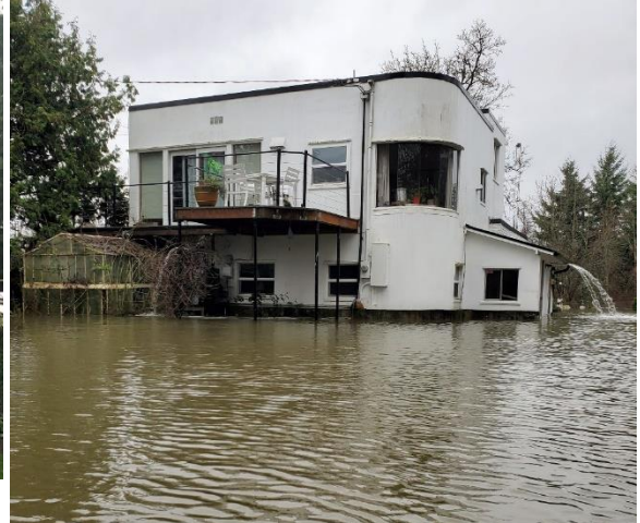
Figure 6.12. Flooding along Clarks Creek December 2015
