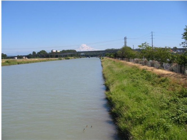
Figure 6.8. Left Bank Levee at Tacoma Wastewater Treatment Plant (looking upstream)
