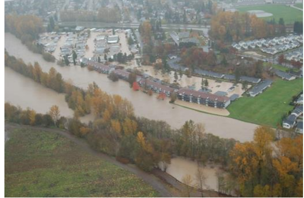
Figure 6.26. Flooding November 7, 2006, Rainier Manor Mobile Home Park, River Grove Apartments, Riverwalk Condos
