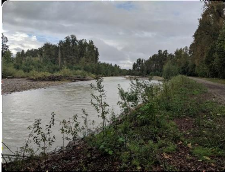
Figure 6.46. Existing Jones Levee looking downstream
