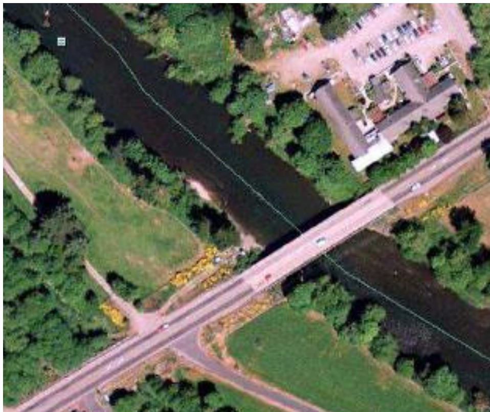
Figure 6.88. SR 507 Bridge and Fresh Start Facility
