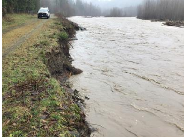
Figure 6.38. Flooding on the Ford Levee, February 7, 2022
