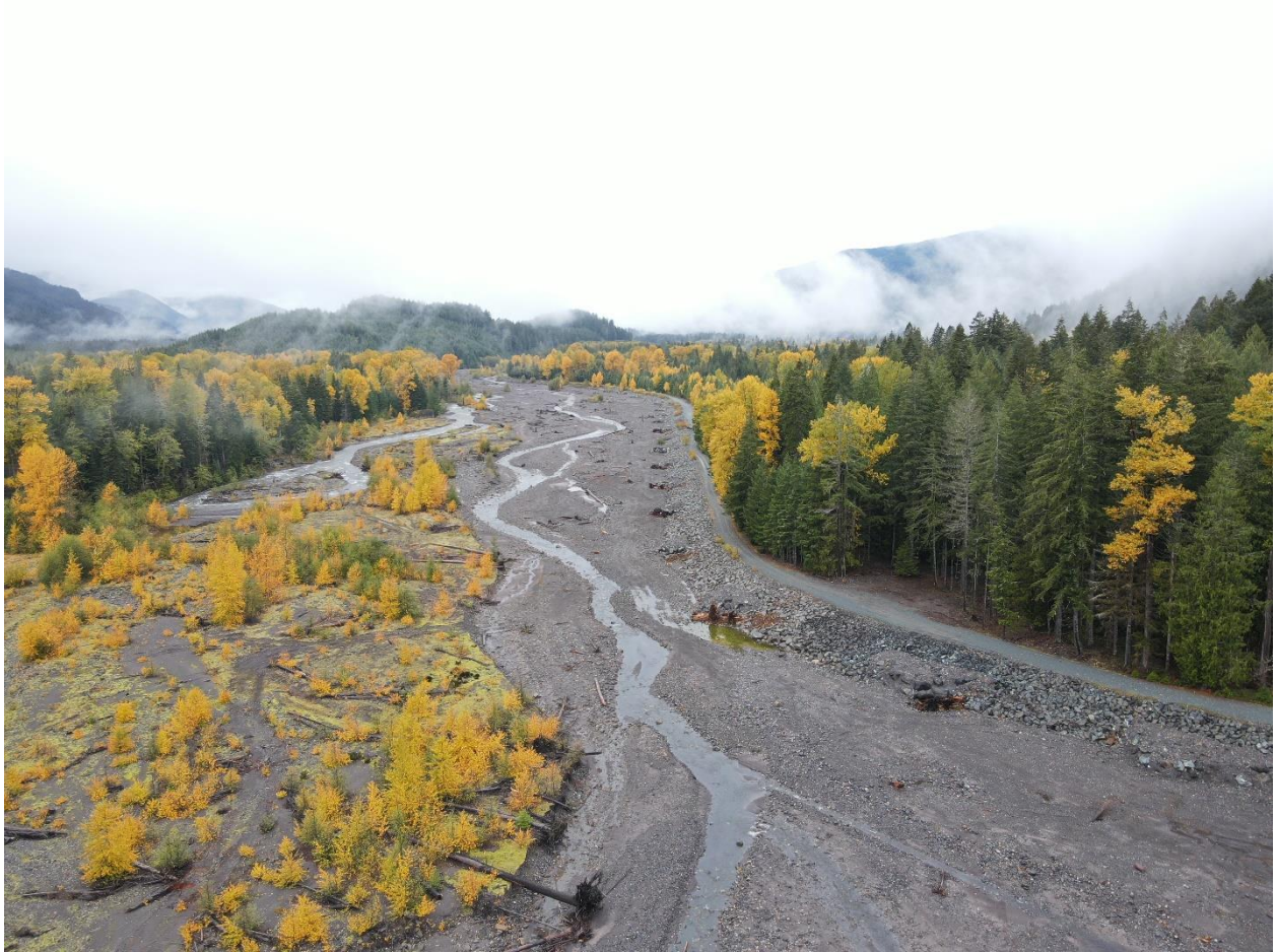
Figure 6.97. Aerial View of the Nisqually Levee Project Showing the Newly Constructed Groins
