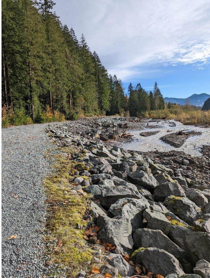
Figure 6.98. A Series of “Groins” Added on the Nisqually Levee
