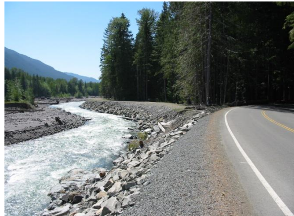
Figure 6.91. Right bank Revetment/Levee near Mount Rainier National Park Entrance Looking Downstream near RM 65.4
