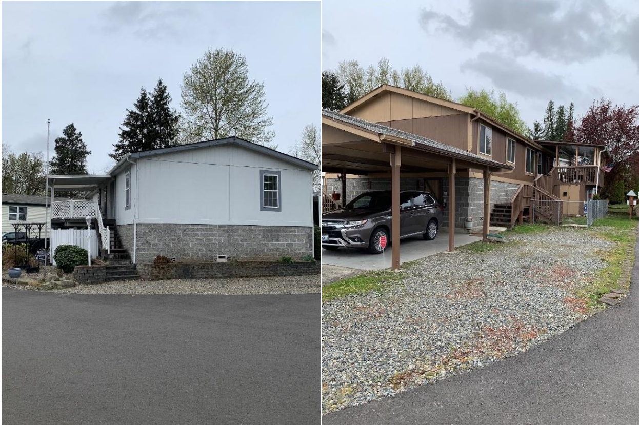
Figure 5.5. Example of a Home Elevation in Sumner, Before and After
