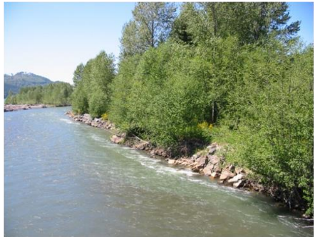
Figure 6.93. Right Bank Armoring Downstream of SR 7 Bridge in Elbe
