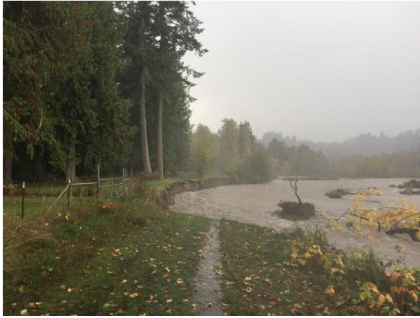
Figure 6.37. Flooding on the Ford Levee, October 22, 2017
