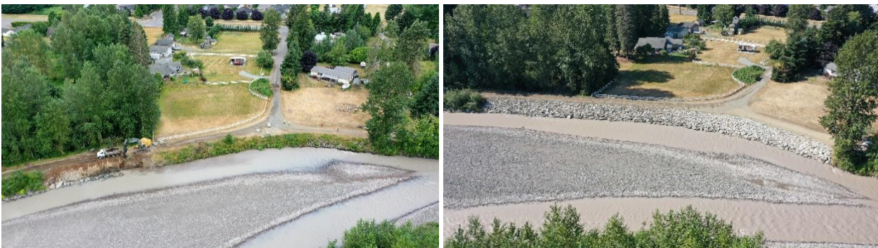
Figure 5.10. Carbon River Left Bank, Milepost 0.4, Before and After 2020 Repair
