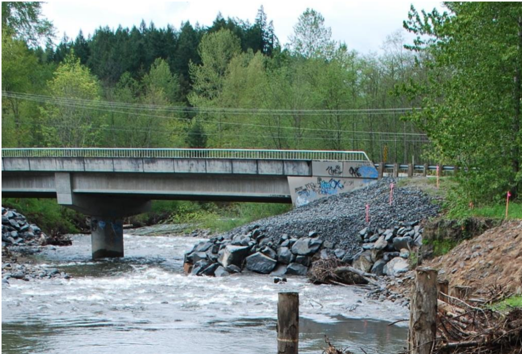
Figure 6.100. Armoring of Bridge Approach at SR 161 Crossing (RM 5.5)
