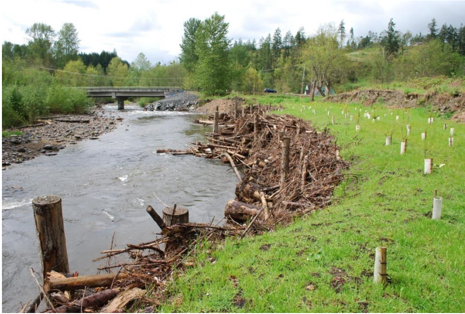
Figure 6.103. Mashel River Restoration Project, Right Bank near RM 5.5
