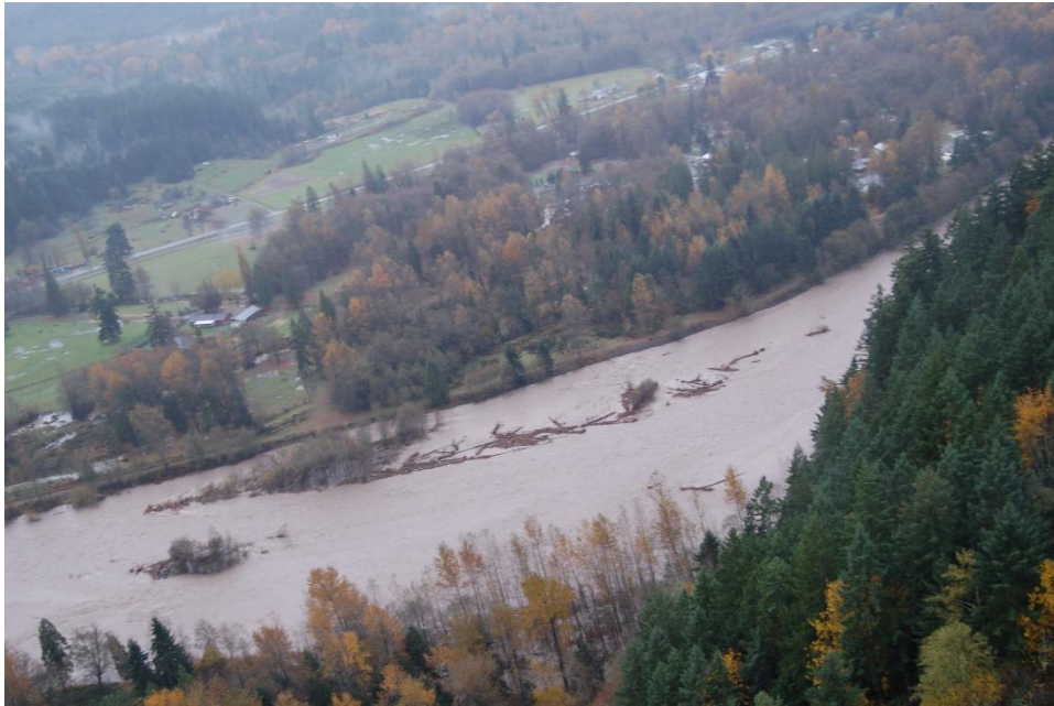
Figure 6.81. Right Bank of Carbon River near RM 5.1
