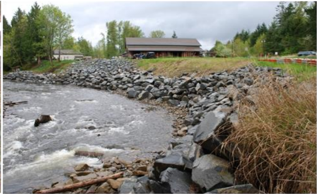
Figure 6.102. Repaired Riprap Bank, RM 5.2–5.3, March 2010
