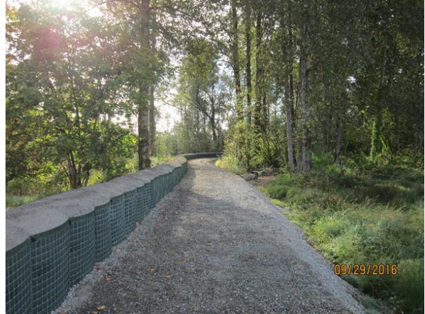
Figure 6.54. Temporary Flood Control Measure, Government Ditch, and the White River, 2016
